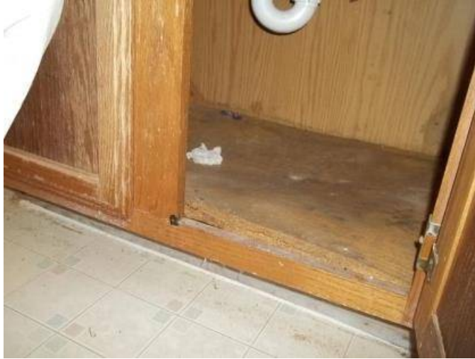
Water damage present to vanity. Possible hidden damage under and behind vanity. Result of ongoing leakage.
