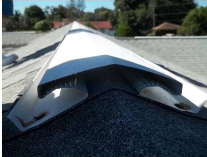
Rusted unsealed nails at ridge vents. The potential for water entry is present.
