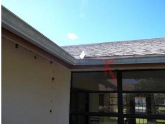
Enclosed patio: The gutter doesn't slope to drain properly.
