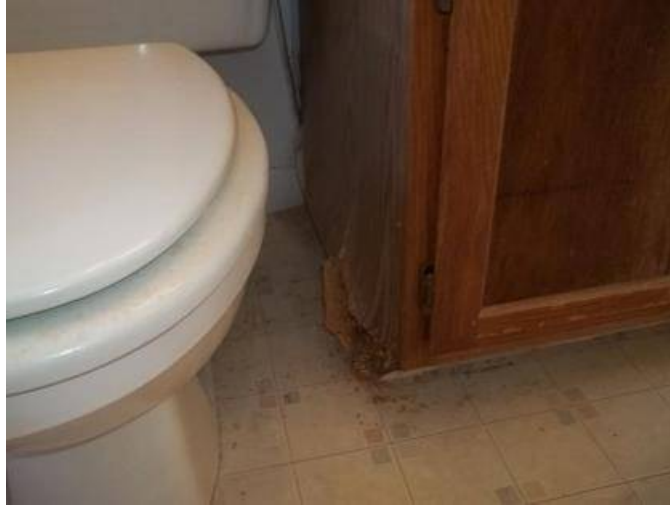
Water damage present to vanity. Possible hidden damage under and behind vanity. Result of ongoing leakage.
