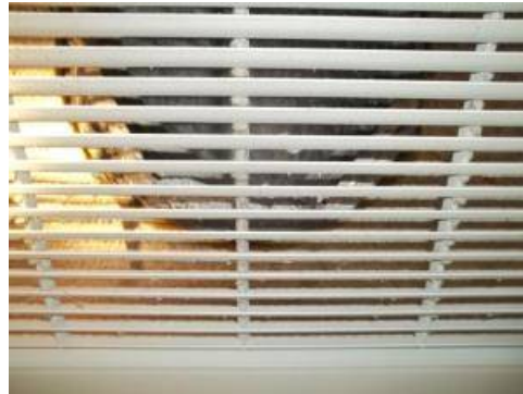
Loose duct connections inside of the return on the hallway ceiling.
