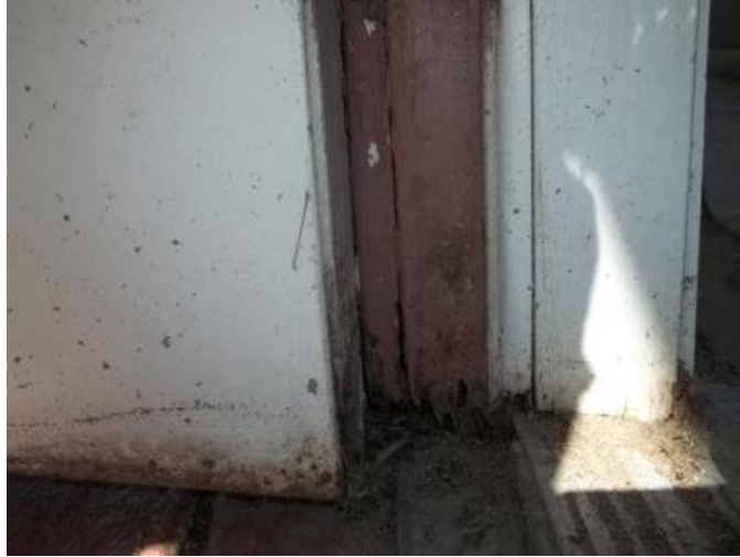
Pedestrian door: Water damage present to structural frame. Wood chord of the door is water damaged.
