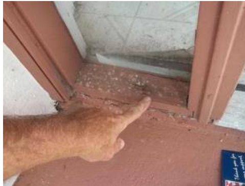
Pedestrian door: Water damage present to structural frame. Wood chord of the door is water damaged.
