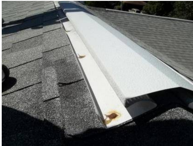
Rusted unsealed nails at ridge vents. The potential for water entry is present.
