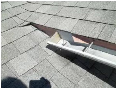
Enclosed patio: The gutter doesn't slope to drain properly.
